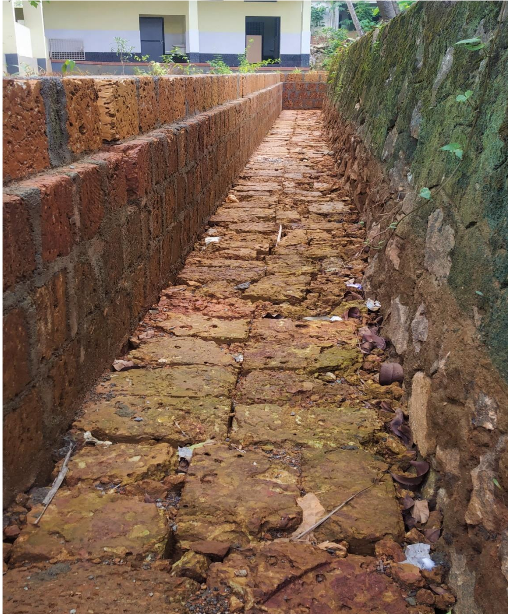
Fig11: Photo of Strom Water Percolation Drain
