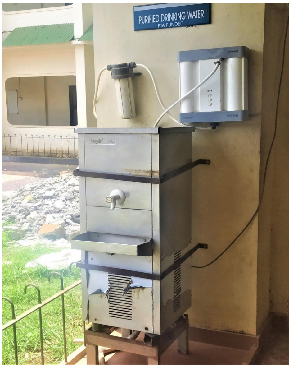
Fig 8: View of Water KIOSK established in the Campus
